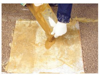
**Step 8.** Turn over the folded wetted mat and pour the remaining resin onto this surface. Spread evenly. Ensure that the resin coats all surfaces and soaks into the matting.
