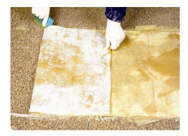
**Step 7.** Fold the mat along the right hand coloured stitch guideline and spread more resin evenly over the mat. Fold along the left hand coloured stitch guideline and spread resin evenly over this surface.
