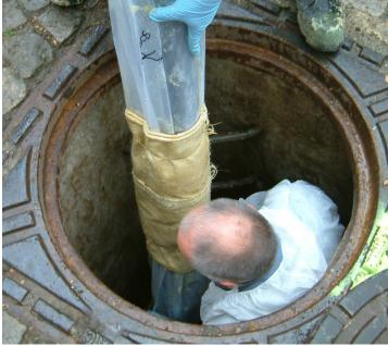
**Step 12.** Attach the flexible adaptor, air push rods and extraction rope to the packer. Ensure all the locking rings are secured against the release mechanism of the quick release air connectors and air push rods.
