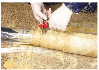
**Step 10.** Roll the fibreglass mat around the packer. Two wire ties are positioned 25mm from the end of the fibreglass mat to secure it. For Radius repairs, a third wire tie is placed at the centre of the mat.
