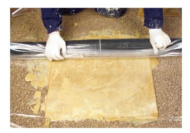
**Step 9.** Position the packer onto the edge of the mat. The folds in the mat should be facing the ends of the packer. Also ensure that the mat is positioned centrally on the packer.
